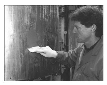
STAINLESS STEEL PUTTY is a stainless steel filled epoxy putty developed specifically for use in repairing stainless steel components, fittings and equipment in hygiene conscious facilities or chemical processing applications. It cures to a non rusting tough inert material that can be easily machined, drilled or tapped to the required tolerances.
