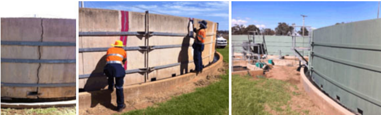
Photograph: Trickle Filter Asset Refurbishment, before (left) during repair (middle) and after application of KIS (right). [Renovasi Trickle Filter Asset, sebelum (kiri), saat perbaikan (tengah), setelah aplikasi KIS (kanan)]
